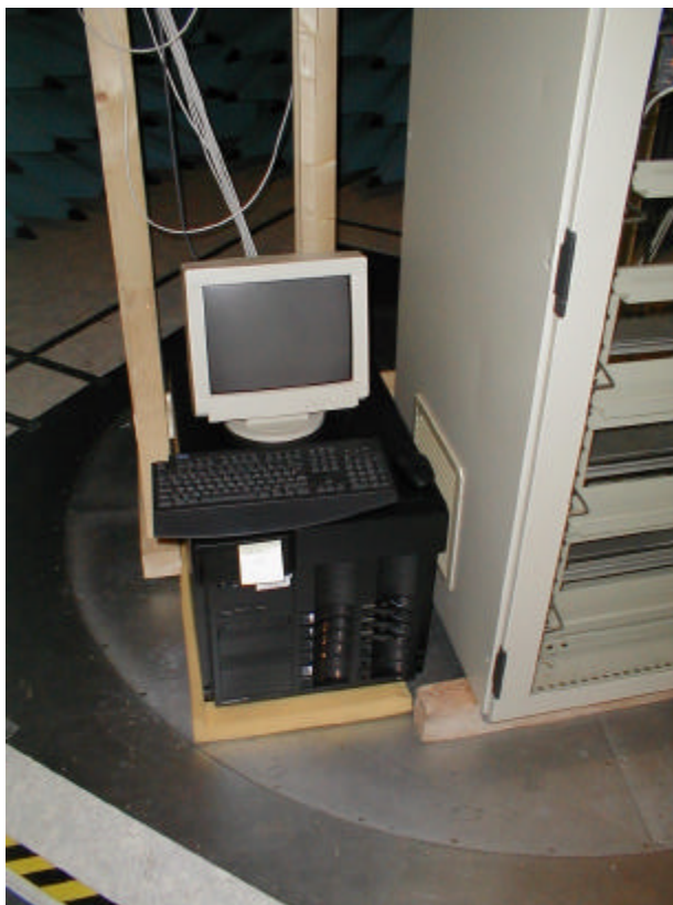
Figure 9: Server 1, front view
